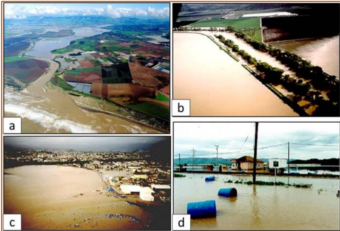
Figure 2-3: Flooding images from 1995 are as follows: (a) 1995 Flooding from Pajaro River (b) 1995 Pajaro River Breached Levee; (c) Aerial view of 1995 Pajaro River Flood; (d) 1995 Pajaro River Flooding.
